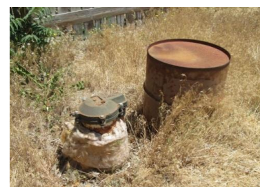
Small public water system wellhead.
