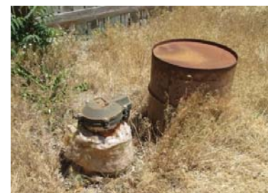
Small public water system wellhead.
