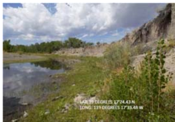
River bank erosion and stabilization.
