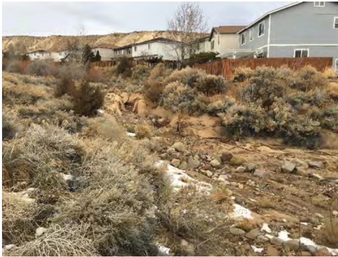
Photo 1, Section 1 above Sapphire Ridge culvert
