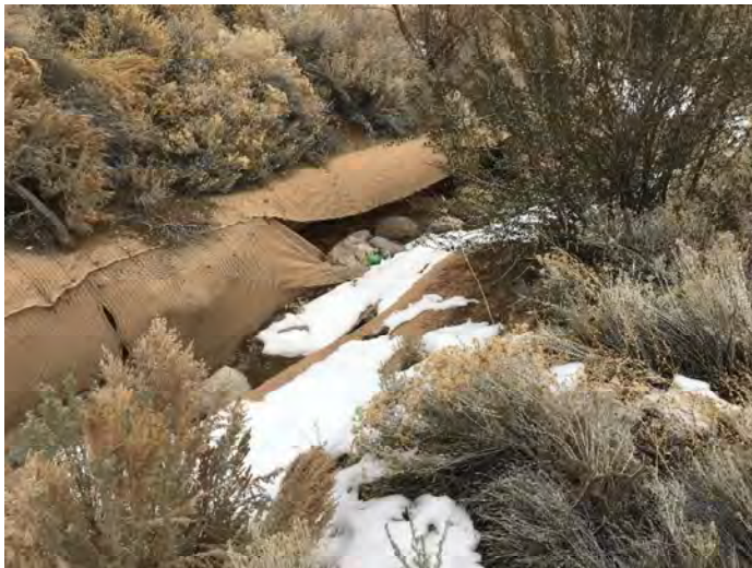
Photo 3, Section 3 below Sapphire Ridge culvert
